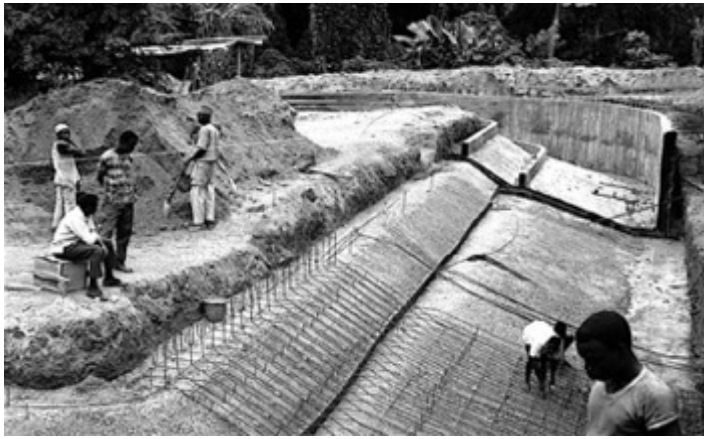
Left: Work in progress in 1969 on the water-filled moat that would form an ape barrier around the outside gorilla and chimp enclosures. Right: Completed ape moat.
